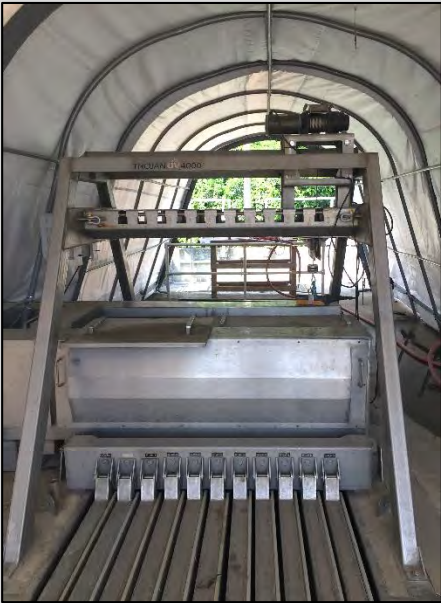
Wastewater Ultra Violet Disinfection Systems Greenway WWTP
