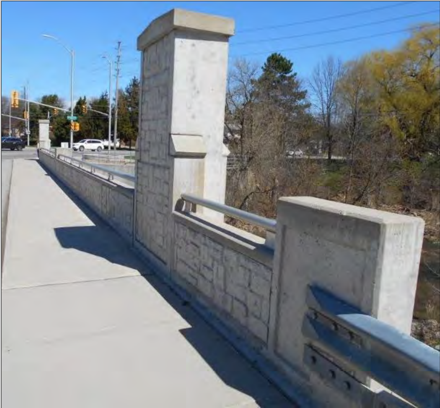
Bridge with Parapet Wall
