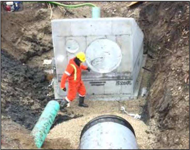
Stormwater Inlet– During Construction
