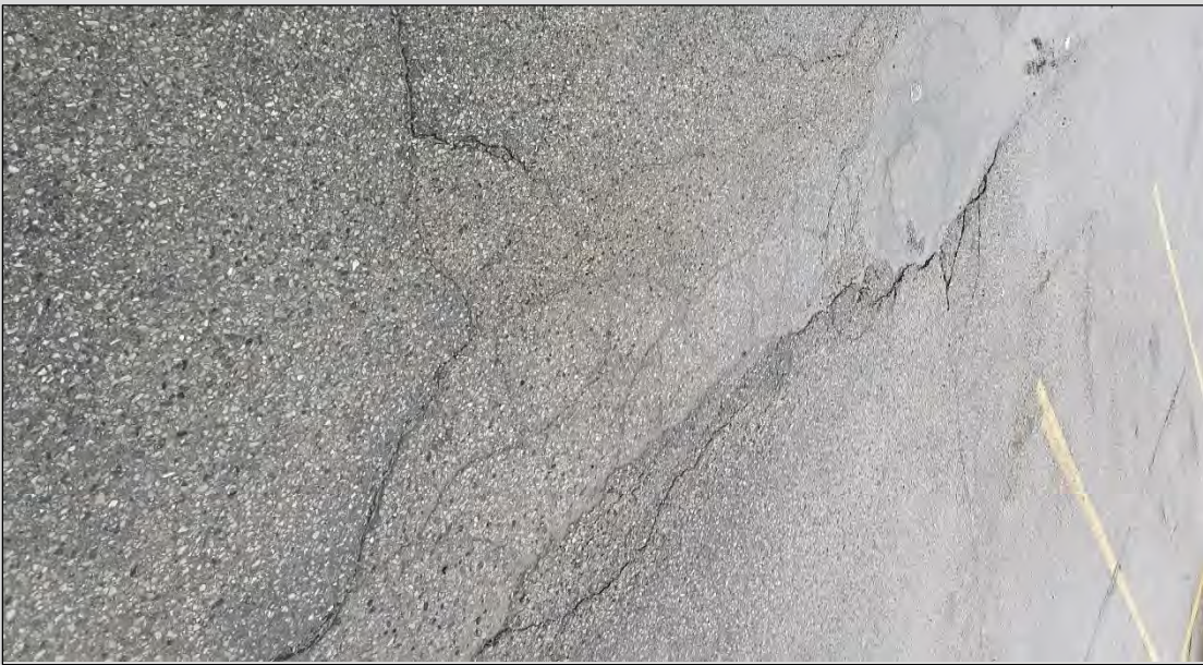
Example of Cracked Surface Lot
