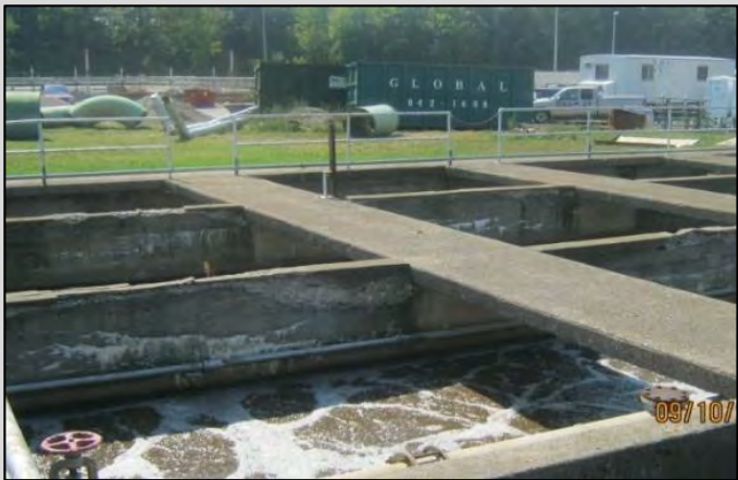
Greenway Section 1 – Crumbling Concrete
