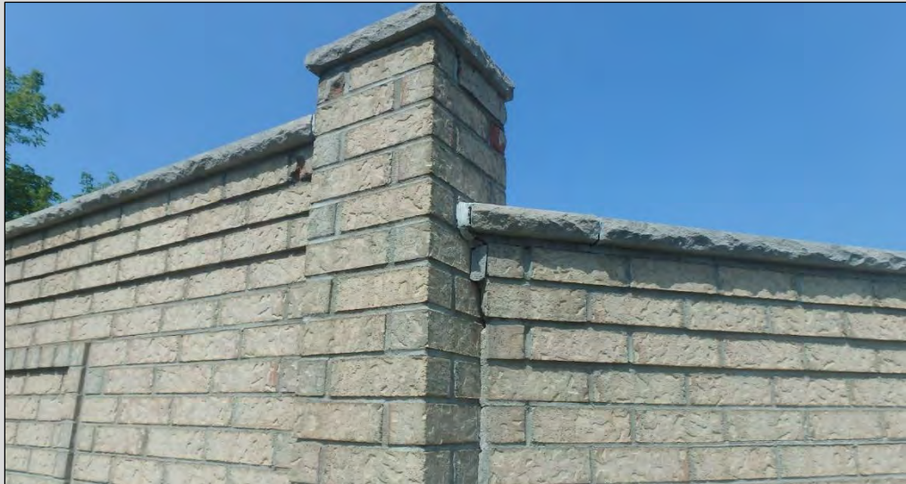
Mason Joints Loss - Noisewall
