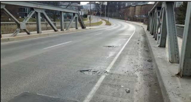
Kensington Bridge – Deck Delaminations
