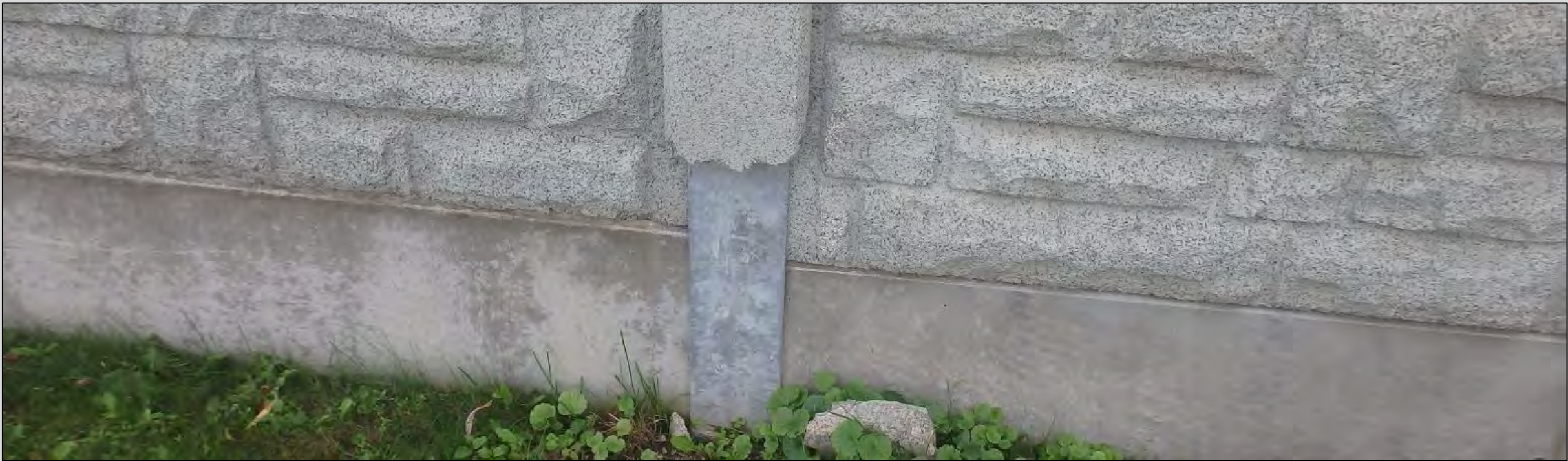
Broken Copping - Noisewall
