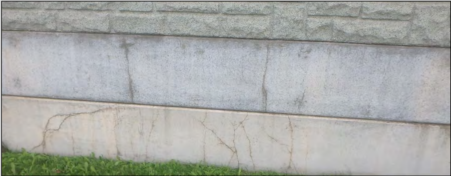
Cracking Retaining Wall
