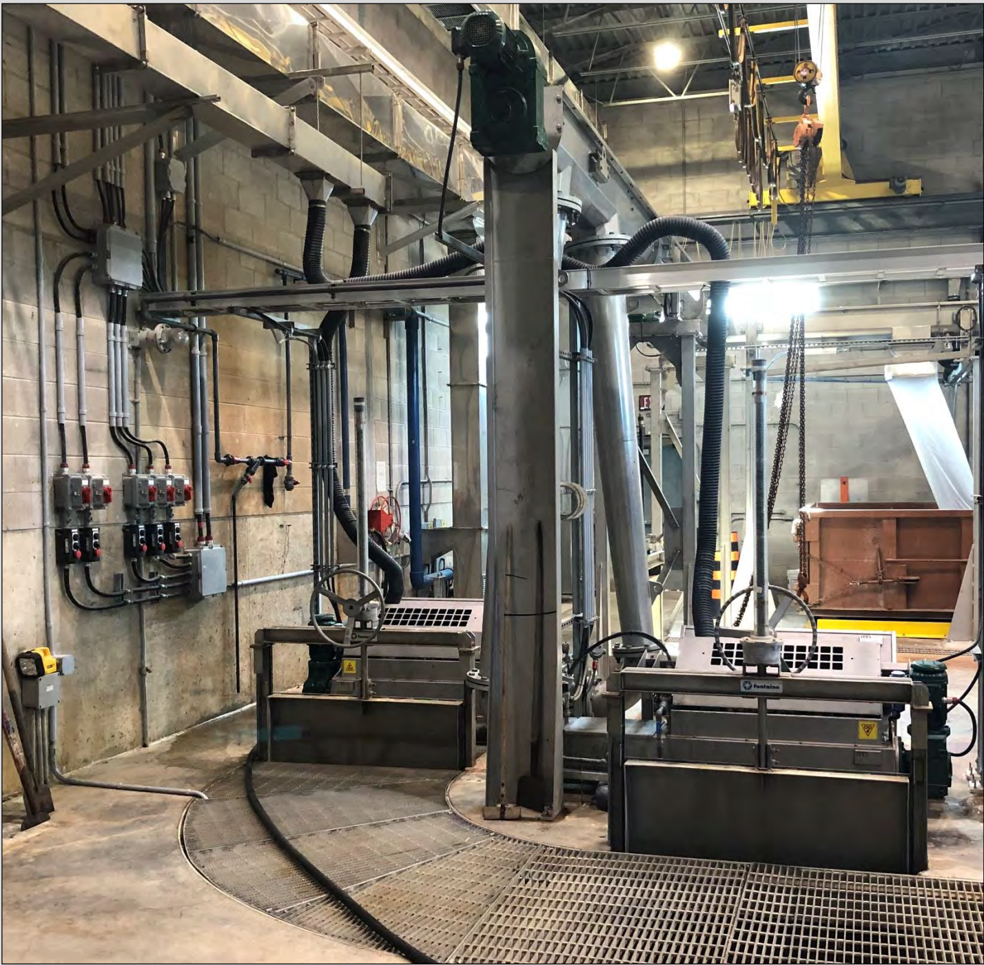
Inlet Screen – Pottersburg Wastewater Treatment Plant
