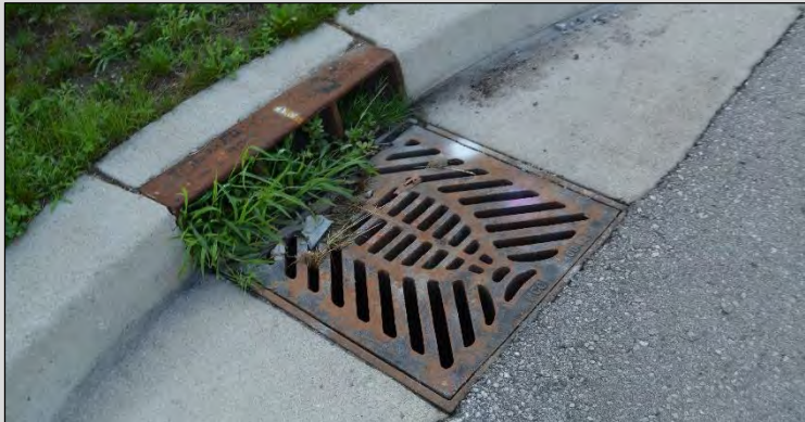
Plants growing in a stormwater Curb Inlet Catch Basins
