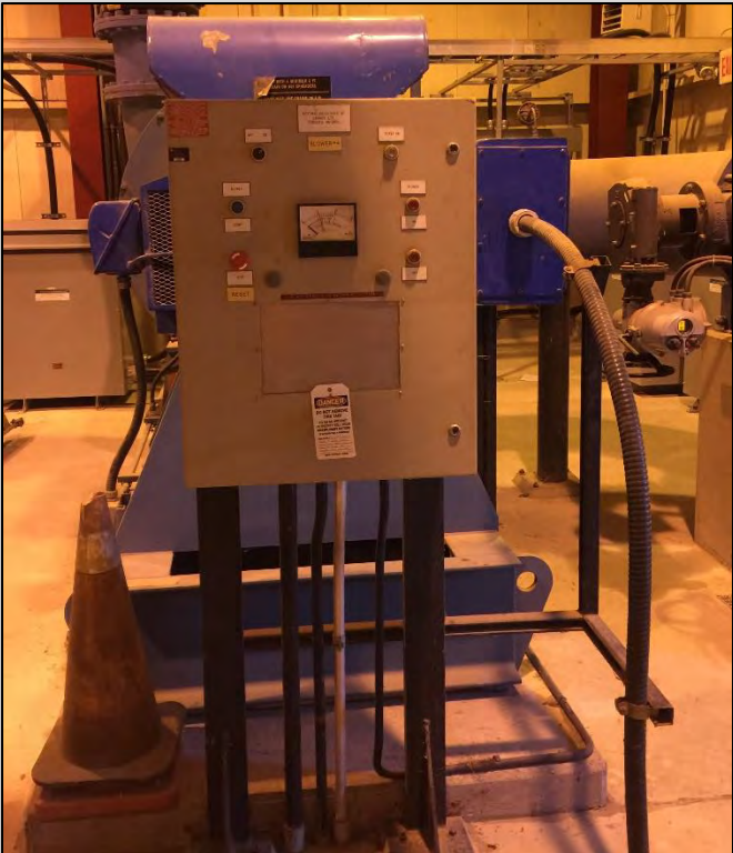
Turbo Blower control unit - Greenway WWTP
