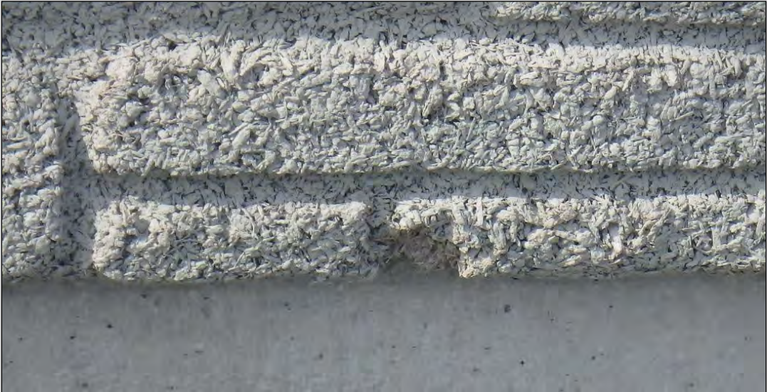
Spalling - Noisewall
