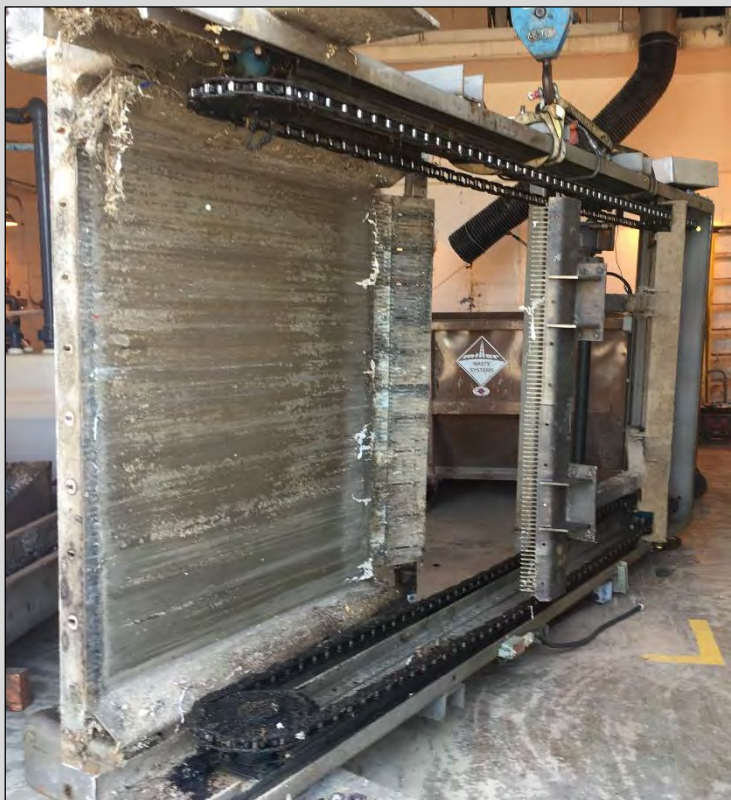
Replaced Screen at Adelaide Wastewater Treatment Plant
