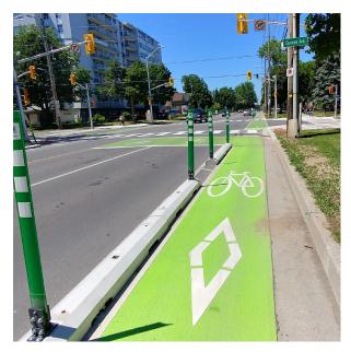
**Cycle track with separation** maintained up to the intersection in London.
