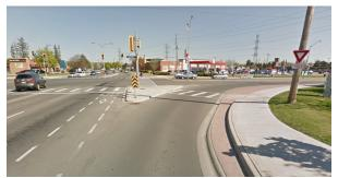
A **truck apron** in Burlington reduces the speed of motor vehicles making a right turn, but still accommodates large trucks.
