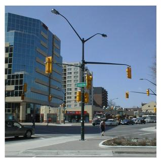
Coordination of pole use to accommodate multiple traffic signal heads and street lighting on a single pole in London.
