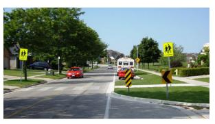
An appropriate motor vehicle **curb radius** is achieved through a curb extension, which also shortens the crossing distance and increases space for green infrastructure.
