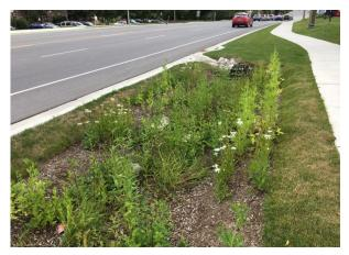
A **rain garden design** that allows stormwater from the road to enter into the depressed area.
