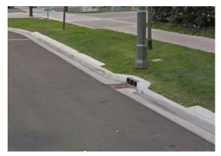
**Catch basin** positioned outside of the wheel path of vehicles and bicycles in London.
