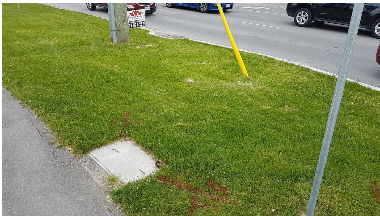
Image 18: Test pitting area showing utility locates for buried electrical cables; facing north at the northwest corner of Adelaide Street and Fanshawe Park Road, June 4, 2019.
