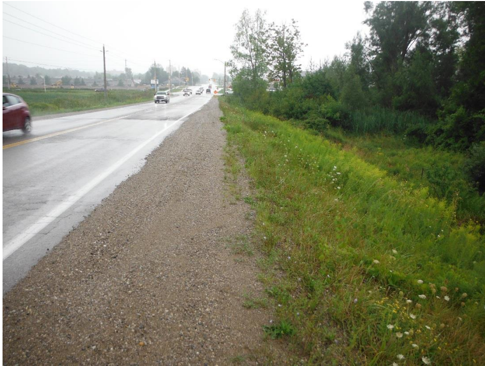
Image 9: A representative example of a sloped area, along with disturbances including Adelaide Street, a drainage ditch, and landscaping; facing south along the western side of Adelaide Street north of Sunningdale Road, August 16, 2018.
