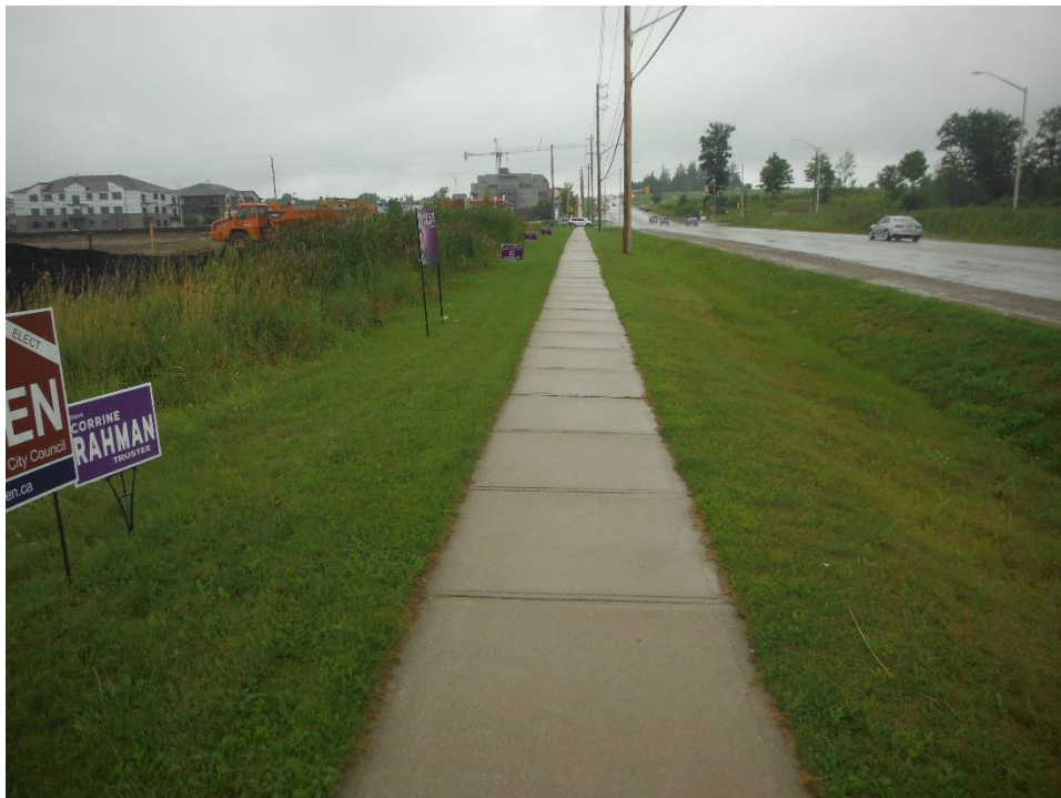
Image 12: A representative example of disturbances including Sunningdale Road, sidewalks, a drainage ditch, buried utilities, and landscaping; facing west along the southern side of Sunningdale Road at the eastern end of the Study Area, August 16, 2018.
