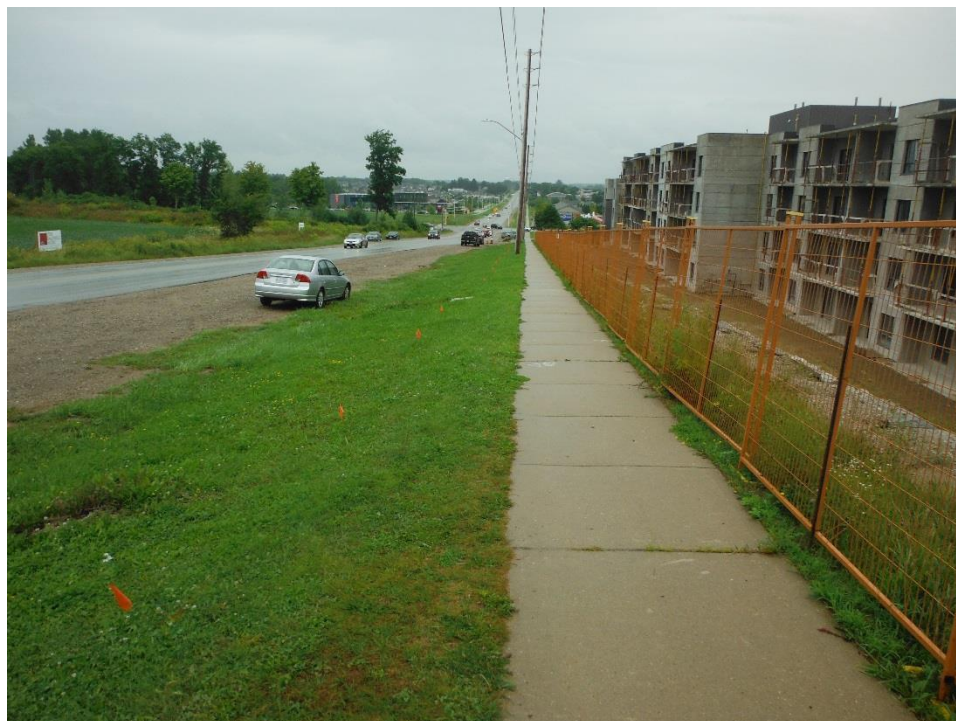
Image 6: A representative example of a sloped area, along with disturbances including Sunningdale Road, sidewalks, buried utilities, and landscaping; facing east along the southern side of Sunningdale Road near Blackwater Drive, August 16, 2018.
