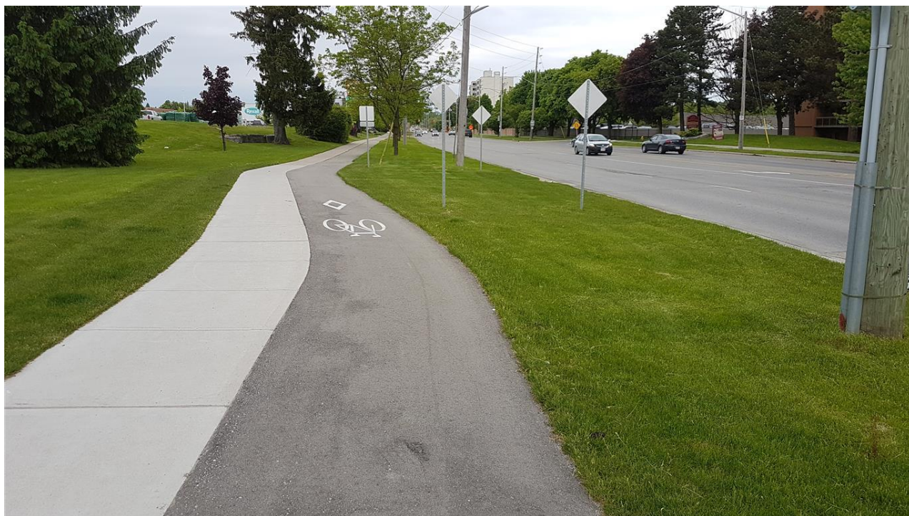
Image 17: Portion of the Study Area identified for test pitting; facing northwest at the northwest corner of Adelaide Street and Fanshawe Park Road, June 4, 2019.
