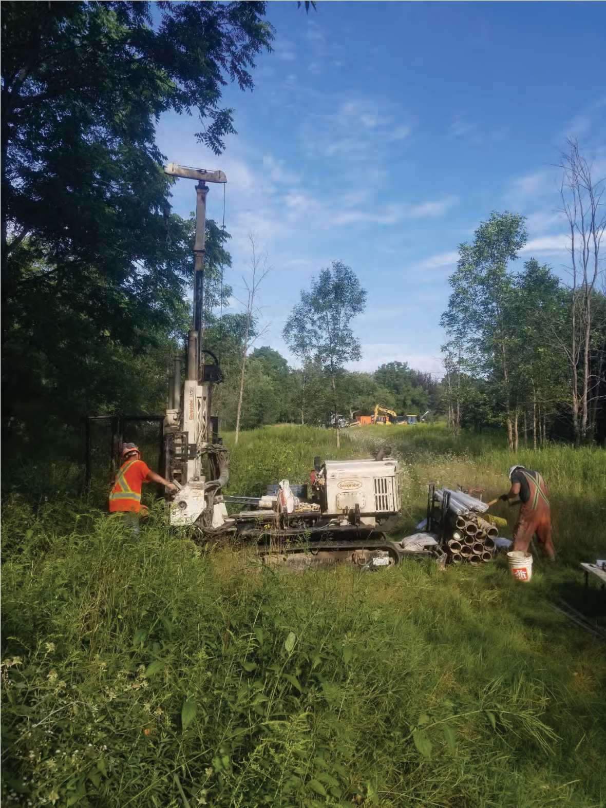
Figure 2 - Drill rig set-up at BH-E18
