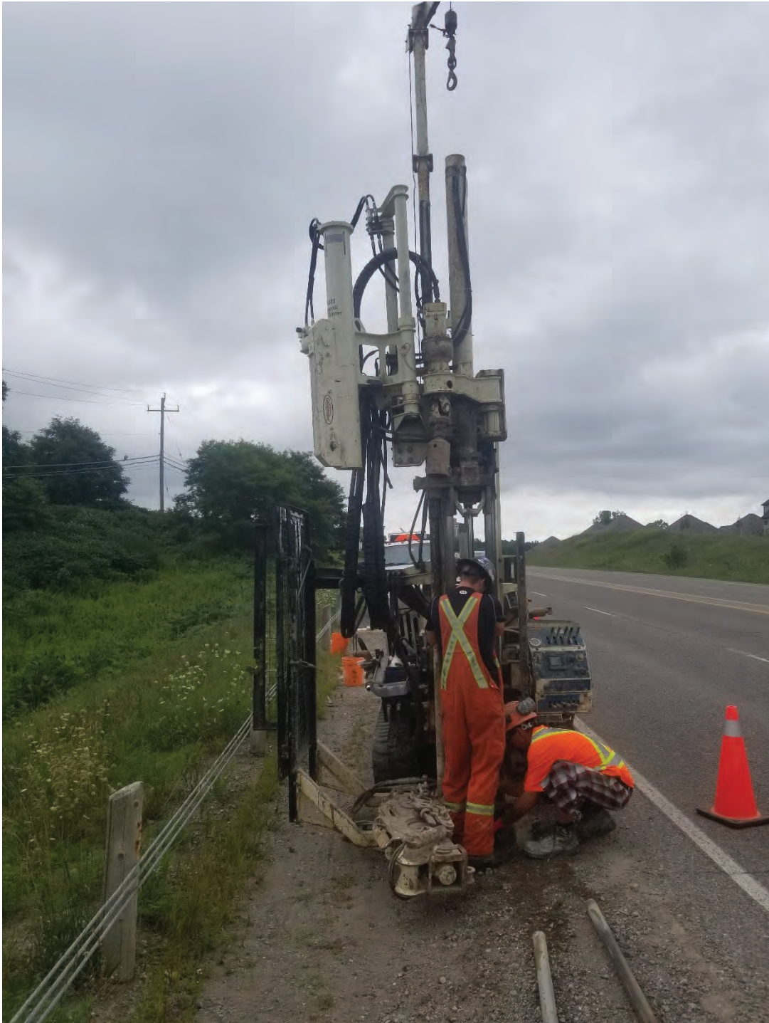
Figure 1 - Drill Rig Set-up on BH-E2
