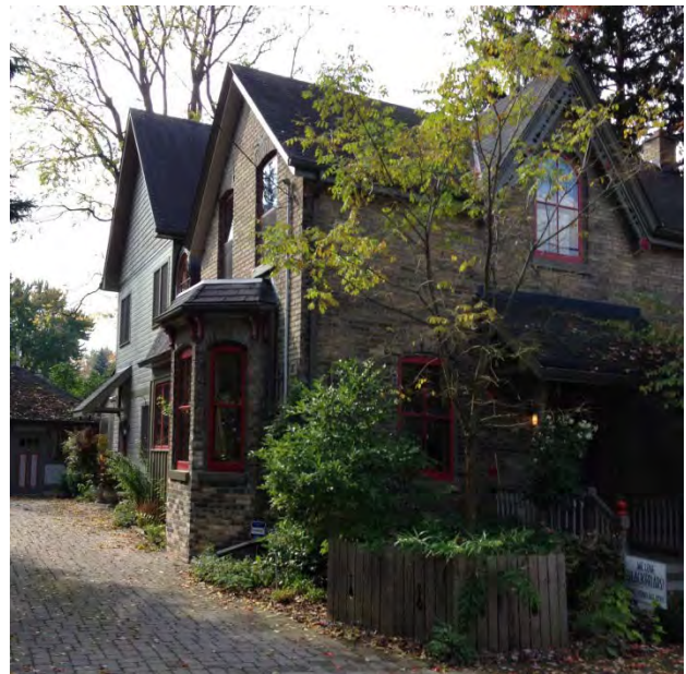
Figure 16: An exterior addition located at the rear of the building and street-facing elevation
