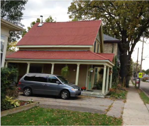
Figure 14: Gable roof with a hipped-roof covered porch
