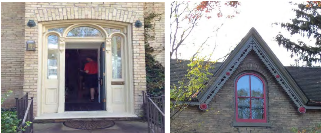
Figure 12: The three-arched, "London" entry door and side lights (left) and 1880s delicate bargeboard and arched dormer window (right).
