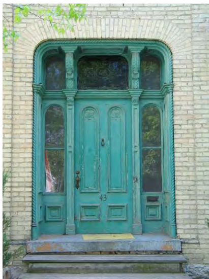
425 Princess Ave.– Door detail
