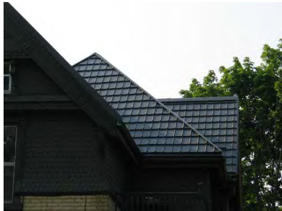
315 Hyman St.– Metal roof shingles
