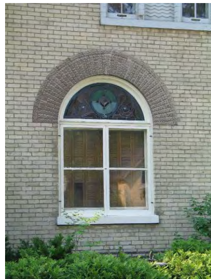
421 Central Ave.– Wood Storm Window
