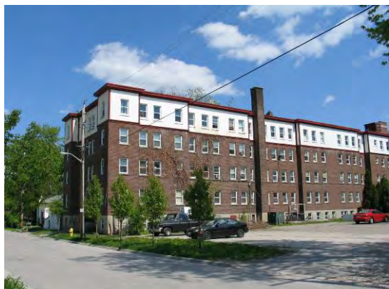
390 Princess Ave.– Stucco fourth floor
