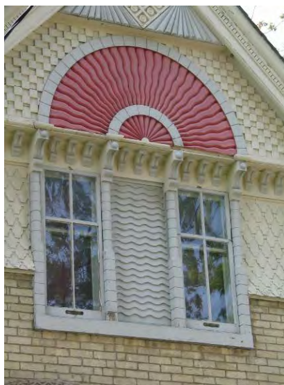
421 Central Ave.– Gable Detail
