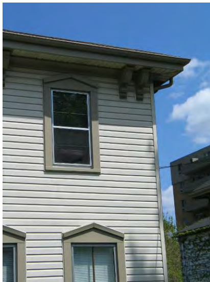
480 Maitland St.– Siding Detail
