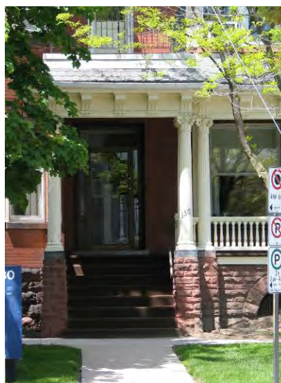
330/332 Queens Ave. – Entrance Detail
