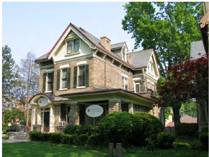
Signage should be based upon design that is contemporary with the building itself.
