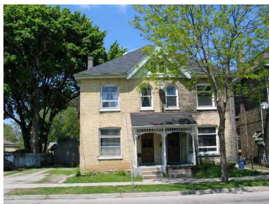
458 Dufferin Ave.– Brick cleaning
