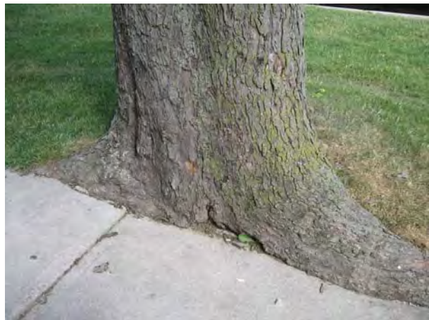
Where tree roots and sidewalks conflict, sidewalks should be re-directed to avoid trunks and roots where possible.
