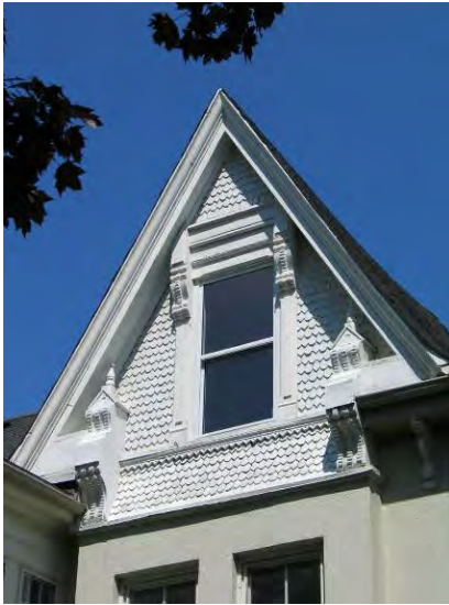
298 Wolfe St.– Gable detail
