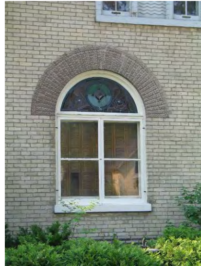
421 Central Ave.– Window Detail
