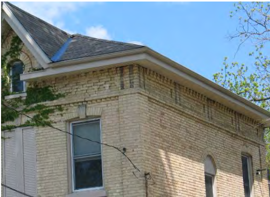
462 Maitland St.– Brackets Removed
