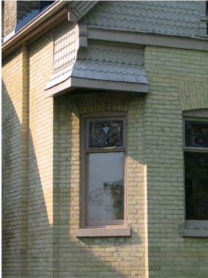
419 Central Ave.– Window detail
