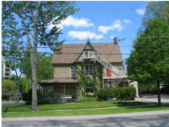
403 Central Ave.— Exposed Fire Escape on Principal
