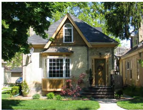
312 Hyman St. – wood trim repair
