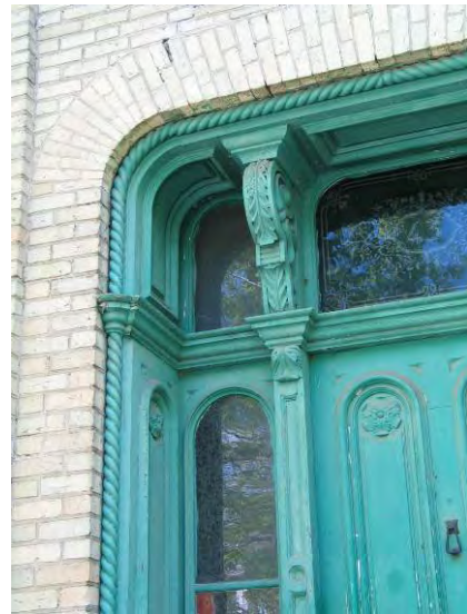
425 Princess Ave. – Window Detail
