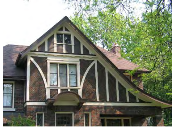
264 Central Ave.– Gable detail
