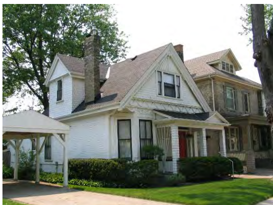
489 Dufferin Ave. – Porch Detail
