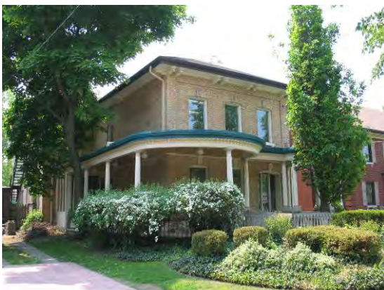
361 Dufferin Ave. – Projecting curved porch
