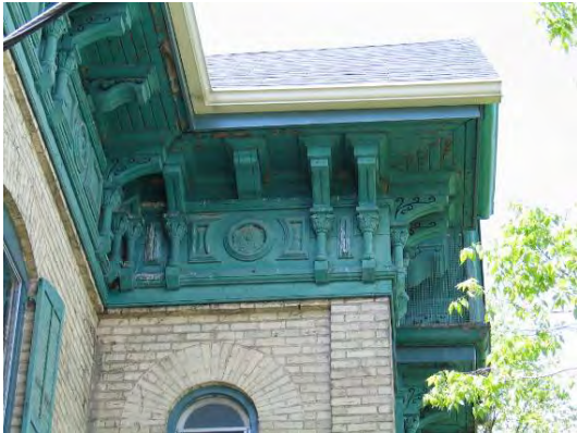
425 Princess Ave.– Soffit detail
