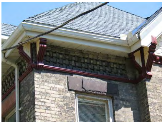
300 Wolfe St.– Brick corbel fascia
