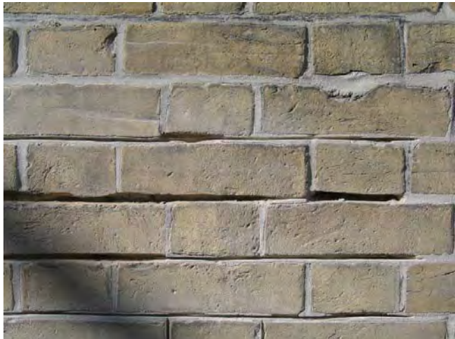
Repointing in Progress
