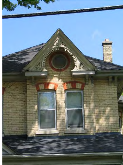
474 Maitland St.– Gable Detail
