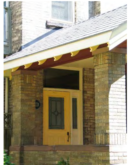
300 Wolfe St. – Porch Detail
