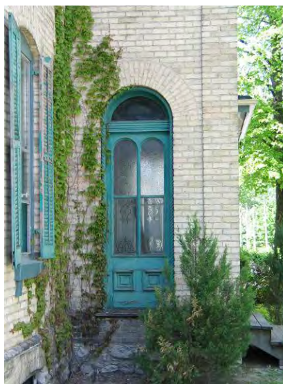
425 Princess Ave.- Window Detail
