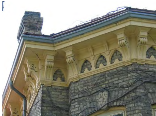
484 Colborne St. – Detail of eave brackets
