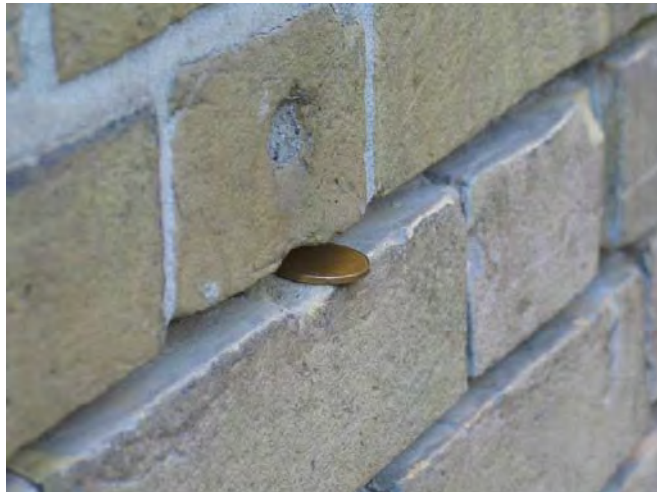
Old mortar cut to depth of loonie prior to repointing
