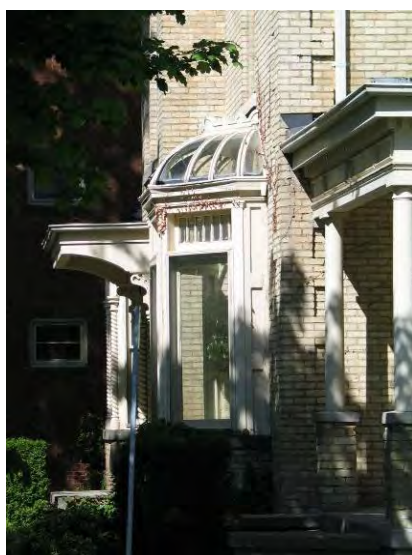
300 Queens Ave. – Glass Roof Window
