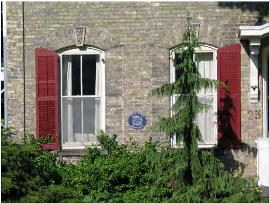
23 Peter St. – Shutter repair
