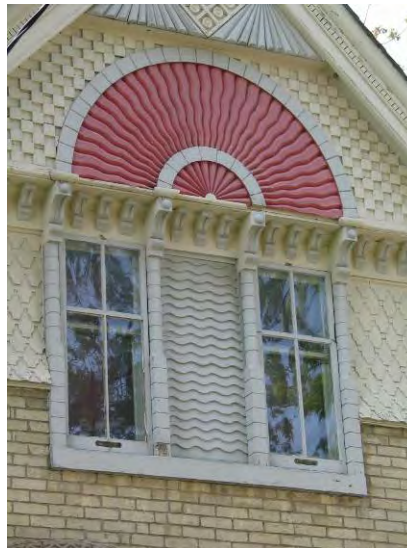
421 Central Ave.– Window detail
