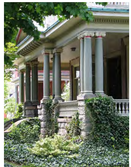
370 Queens Ave.– Porch Detail
