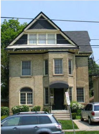
628 Wellington St. – Modern Awning
