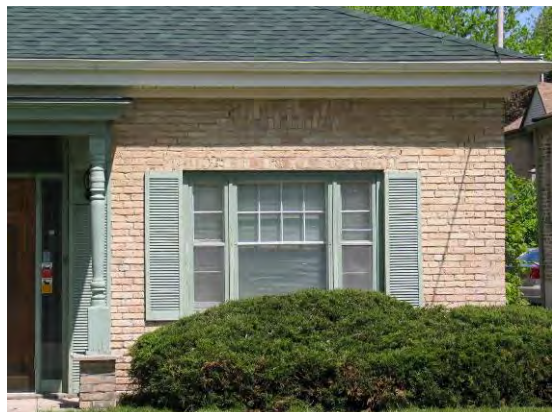
28 Cartwright St. – Mis-sized shutter detail
