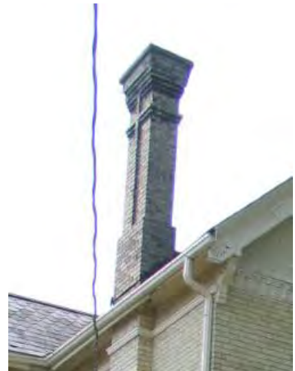
303 Wolfe St.– 1893 High Victorian, Chimney detail
