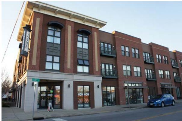
Example of contemporary 3 storey mixed-use development with contemporary architectural details.
