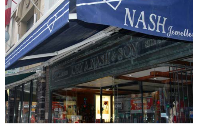
Awnings providing shelter over main entranceways in Downtown London, ON
