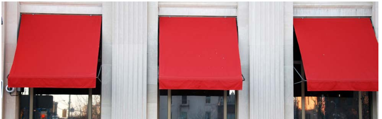
Awnings installed in Downtown London, ON
