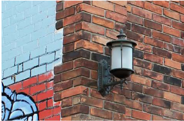
Exterior mounted light fixtures in Old East Village, London, ON
