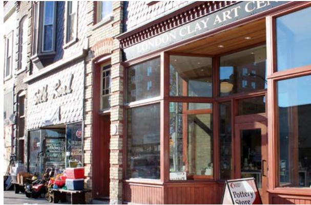
Minimized height of sign band to maximize the size of display windows, London, ON
