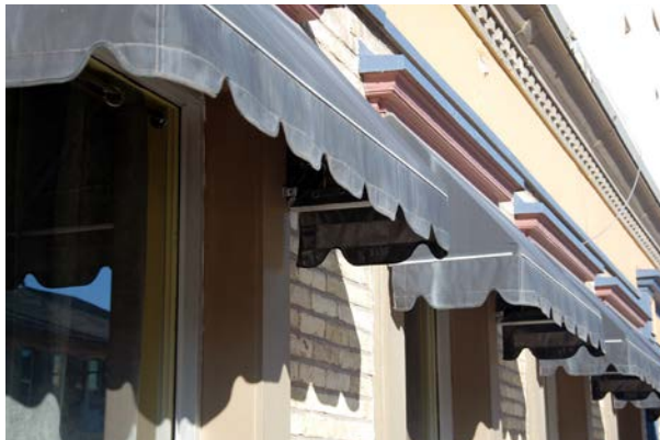
Consistent size, profile and location of awnings in Old East Village, London, ON
