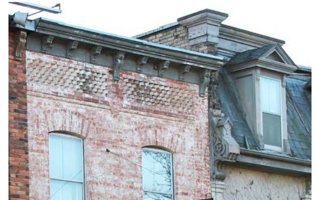
Cornice details in Old East Village, London, ON
