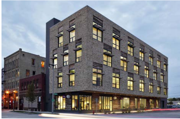
Example of contemporary 4 storey mixed-use development lining up floor heights and horizontal datum lines.
