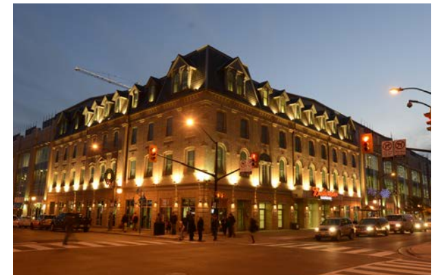
Up-lighting in Downtown London, ON
