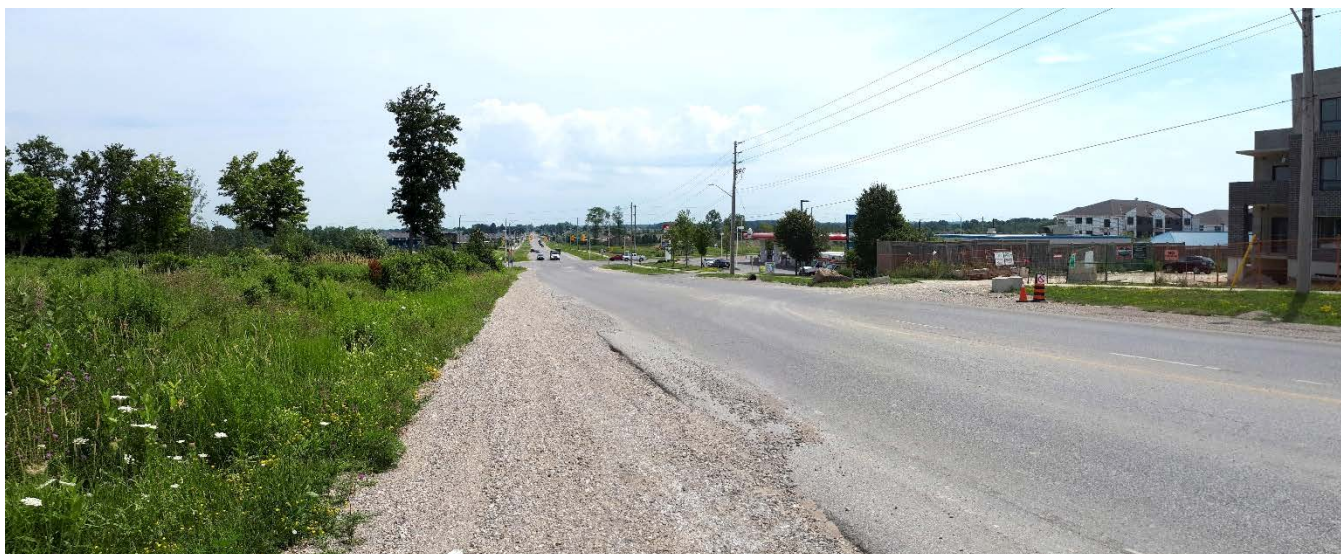
Figure 13: View east towards the north intersection from the edge of 660 Sunningdale Road East (July 20, 2018).
