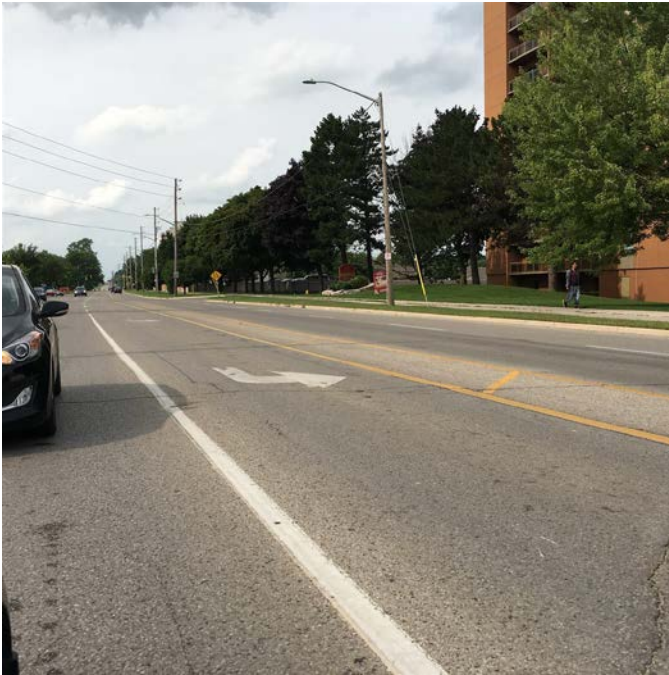
Photograph 7: Adelaide Street North, just north of Fanshawe Park Road, looking north.
