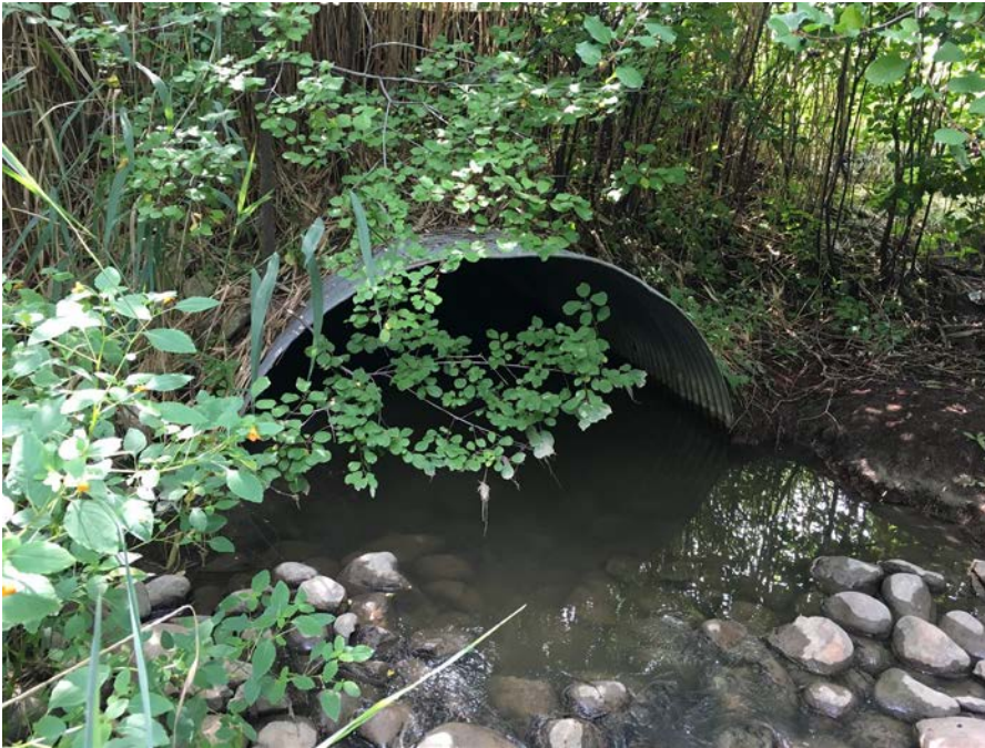
Photograph 11: Section A-A', Stoney Creek Valley North, looking west at CSP outlet.
