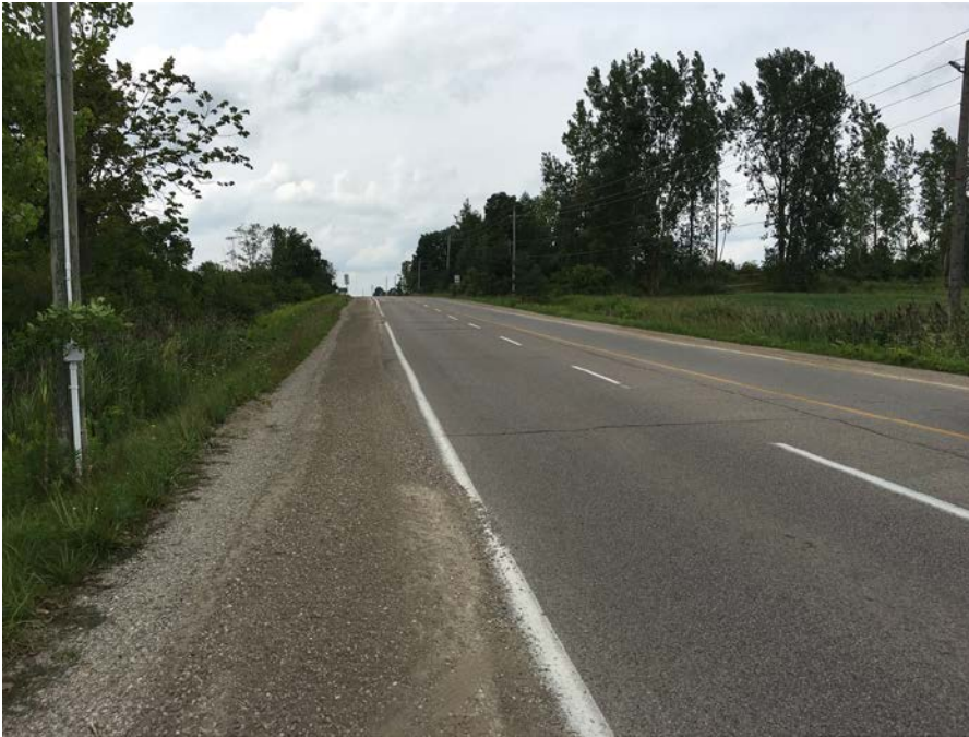
Photograph 1: Adelaide Street North looking north at north limit of site.
