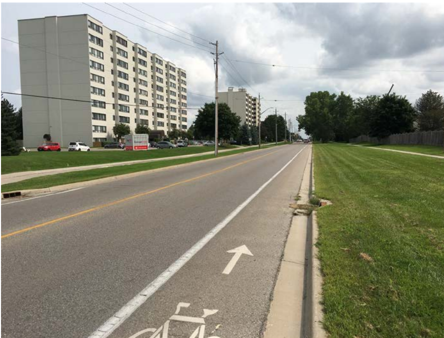
Photograph 6: Adelaide Street North looking south at Stoney Creek Valley North crossing. Note wide boulevard.
