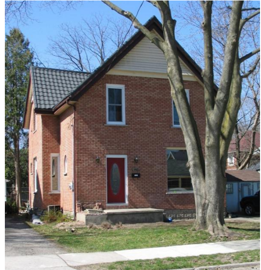
Image 23 - Rebuilt residential, 107 Marley
