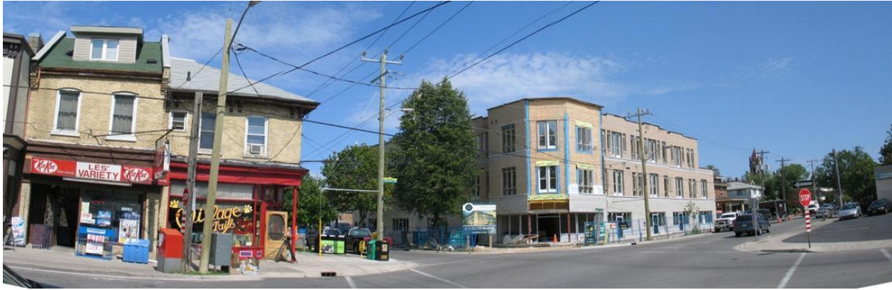
Image 24 - New Commercial Building, 162 Wortley
