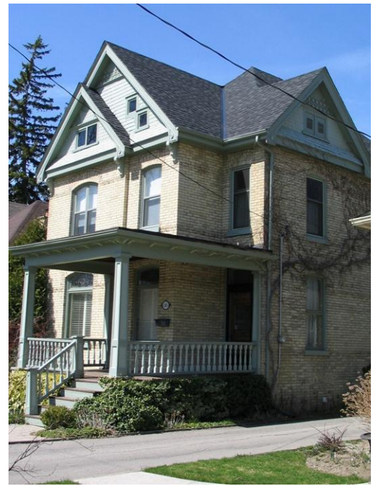
Image 15 - Gabled roof, 86 Elmwood
