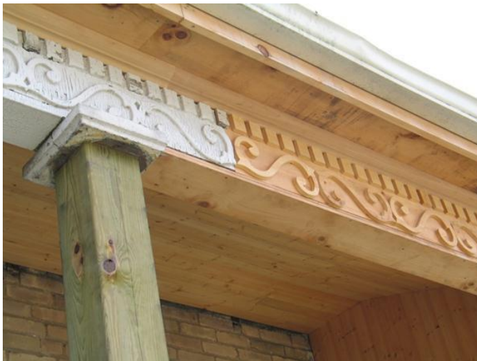
Image 29 - Fascia repair detail, 17 Elmwood
