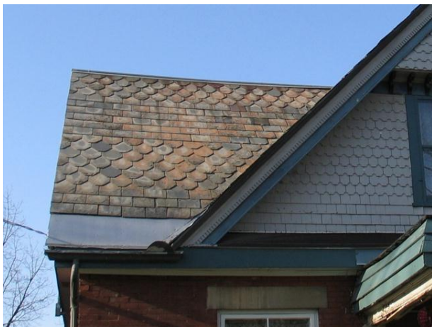
Image 30 - Roofing slates, 88 Duchess
