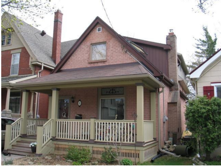
Image 22 - Rebuilt residential, 15 Victor
