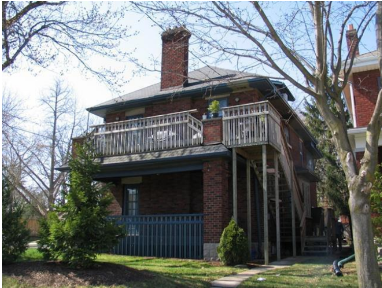
Image 18 - Balcony alteration, 197 Ridout, replication of baluster texture and new stair in unobtrusive location.
